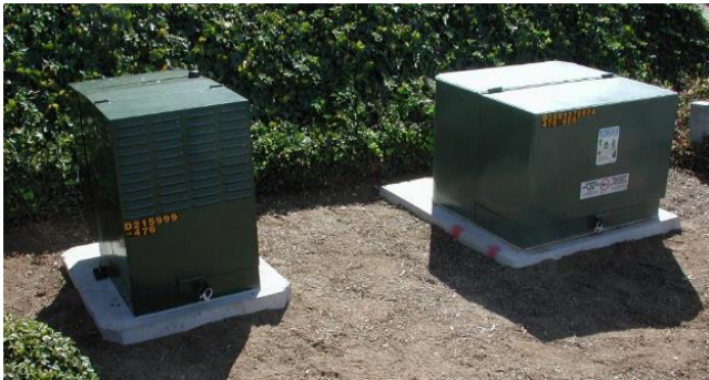
IPR-50 (left) adds distributed, dynamic power control to the existing pad-mounted transformer(s)
